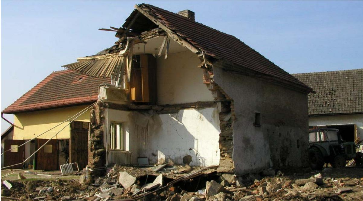
Figure 3. Failure of a structure without ring beams.
