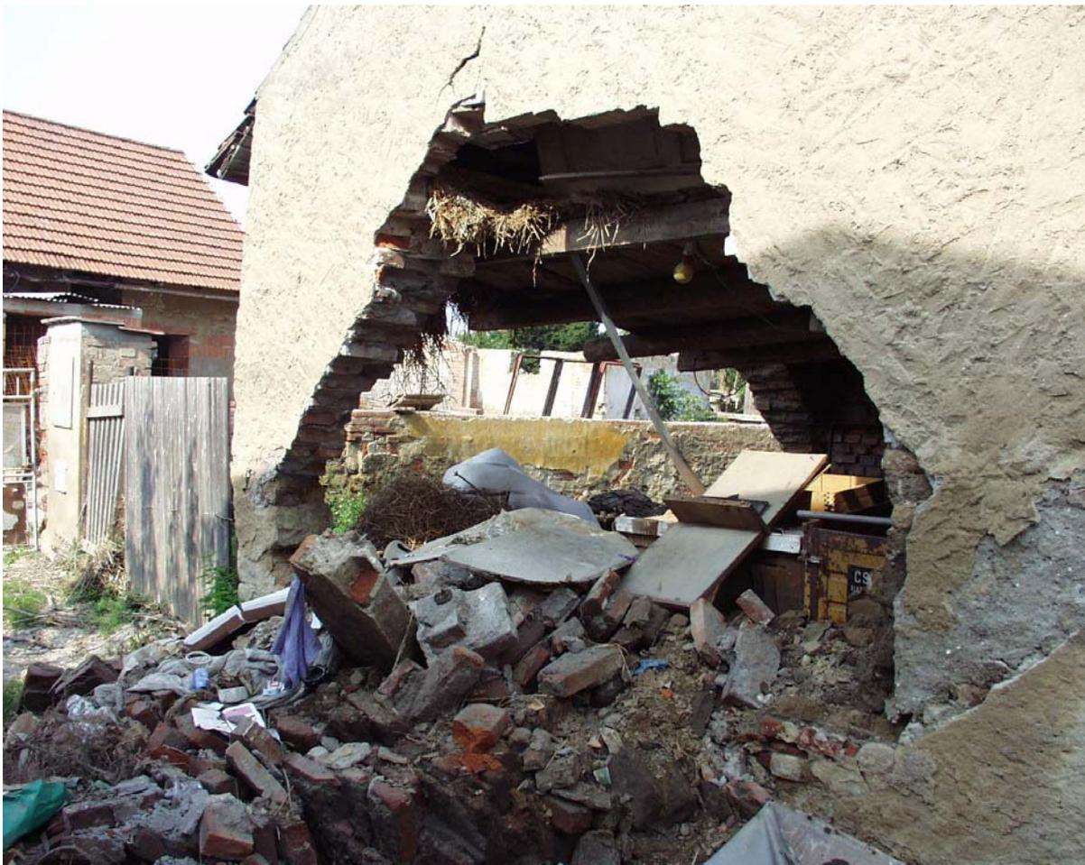
Figure 4. Failure of a structure with unfired masonry units.
