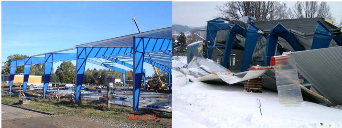
a) under construction
