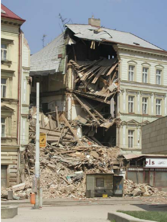
a) undermined foundations
