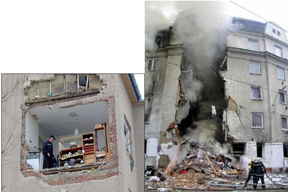
Figure 6: Failures of structures due to gas explosions
