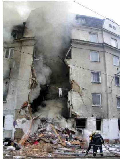
b) progressive collapse
