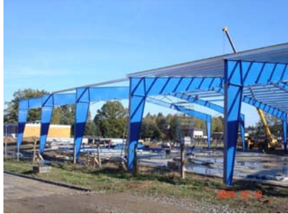
a) under construction
